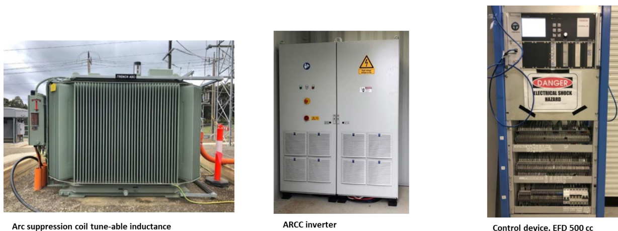
Figure 6: Three components to ARCC technology
