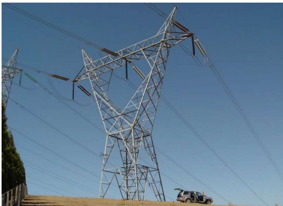
Figure 1: DDTS-SMTS No. 1 330 kV strain tower
