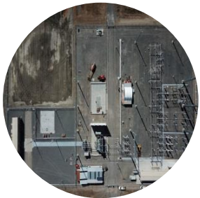
226MW Murra Warra Wind Farm
